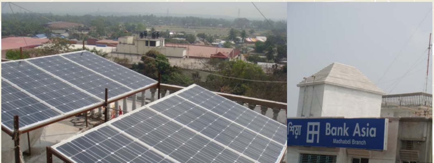
Solar powered Madhabdi Branch of Bank Asia
